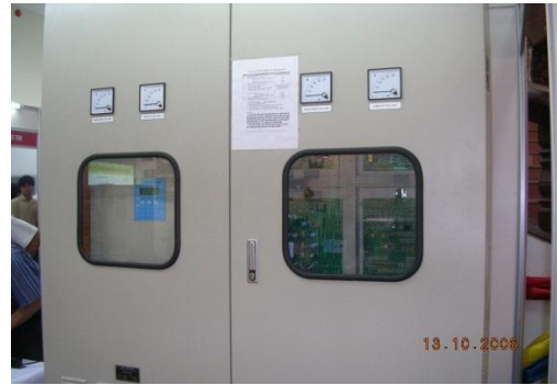
Fig.13. Excitation control cabinet
